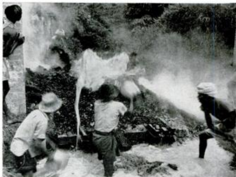
BURNING RAILWAY BRIDGE near Kerdau, set on fire by bandits, is wet down by some rail workers. The derailling of Malaya's few trains is also frequent.
