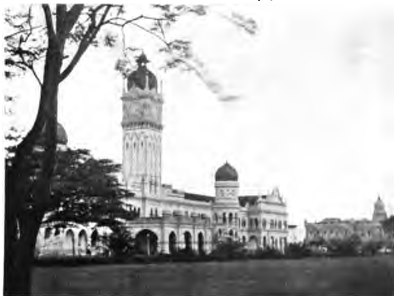
GOVERNMENT OFFICES, KUALA LUMPUR, SELANGOR.
